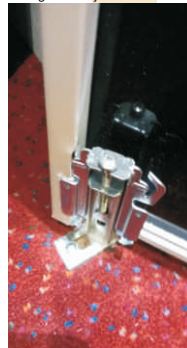
Easy door adjustment via lower door jamb, pivot locator and internal integrated adjustment device
